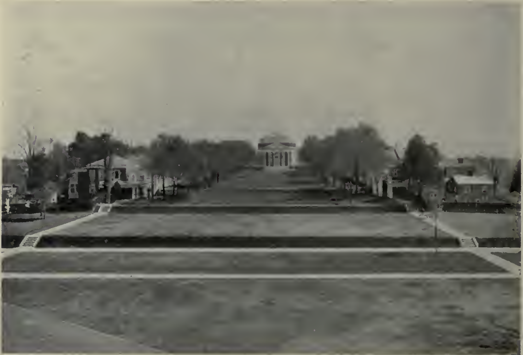
View From Academic Building, of Lawn and South Front of Rotunda.
